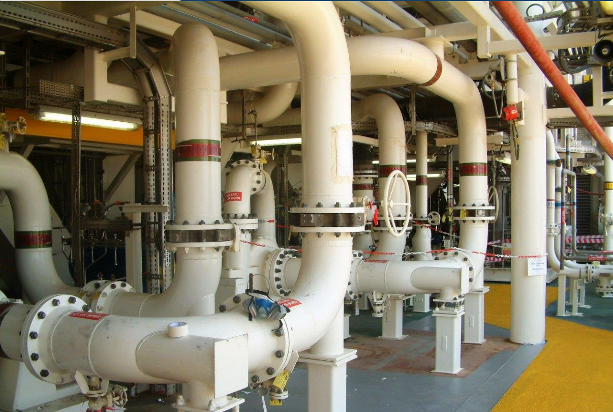
COOLING WATER PIPEWORK COMPLETION
